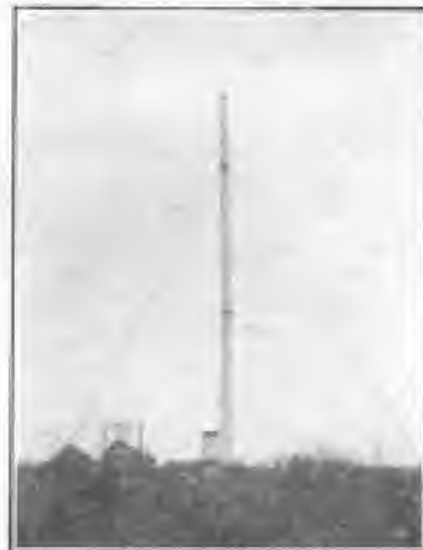
Appreciated Wireless Station near Perth, W.A. Note the Direction Finding Aerial
